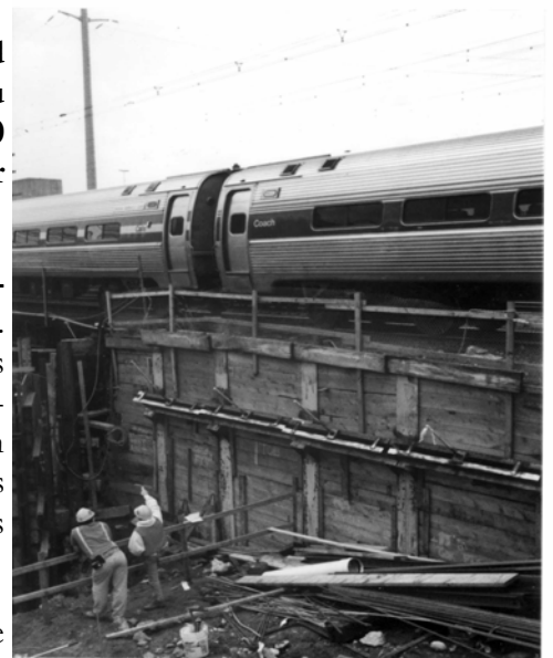
Staged construction: Stamford Railroad Station
