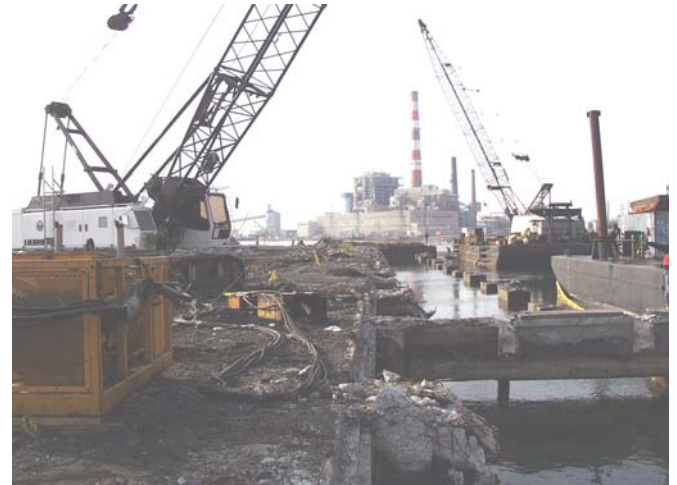
Bulkhead following demolition
